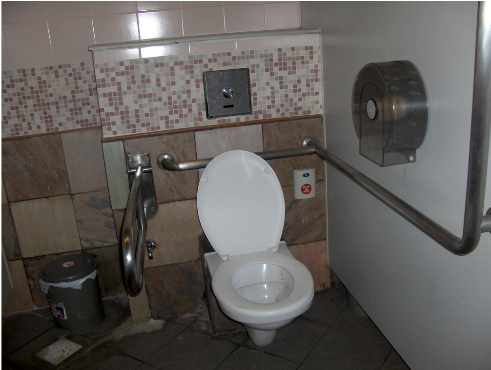
Figure 1i: Female Handicap Toilet - Toilet Bowl, Support Handrail, Toilet Roll Dispenser, Automatic Flush, Sanitary Bin
