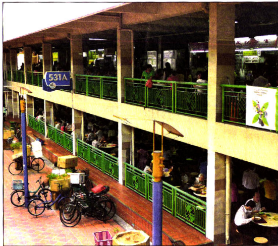
The 31-year-old Hong Lim Market and Food Centre will be given wider passageways and improved access for the elderly and the handicapped. Its toilets will also be improved. PHOTO: LIANHE ZAOBAO
