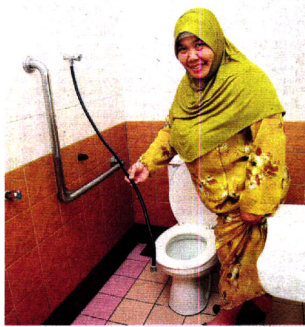
Dr Asiah Abdul Rahim showing the design of the hose which does not touch the ground in a toilet at the International Islamic University.
